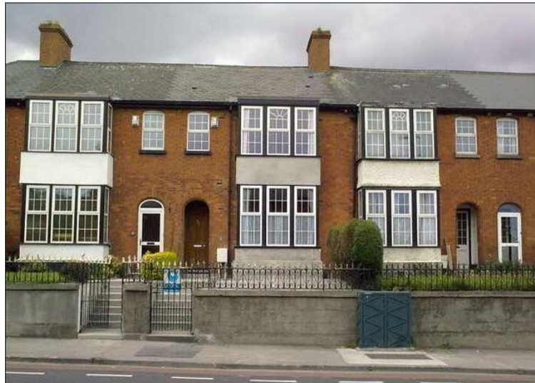
Figure 8 Properties on Botanic Road (Note steps to entrances)
